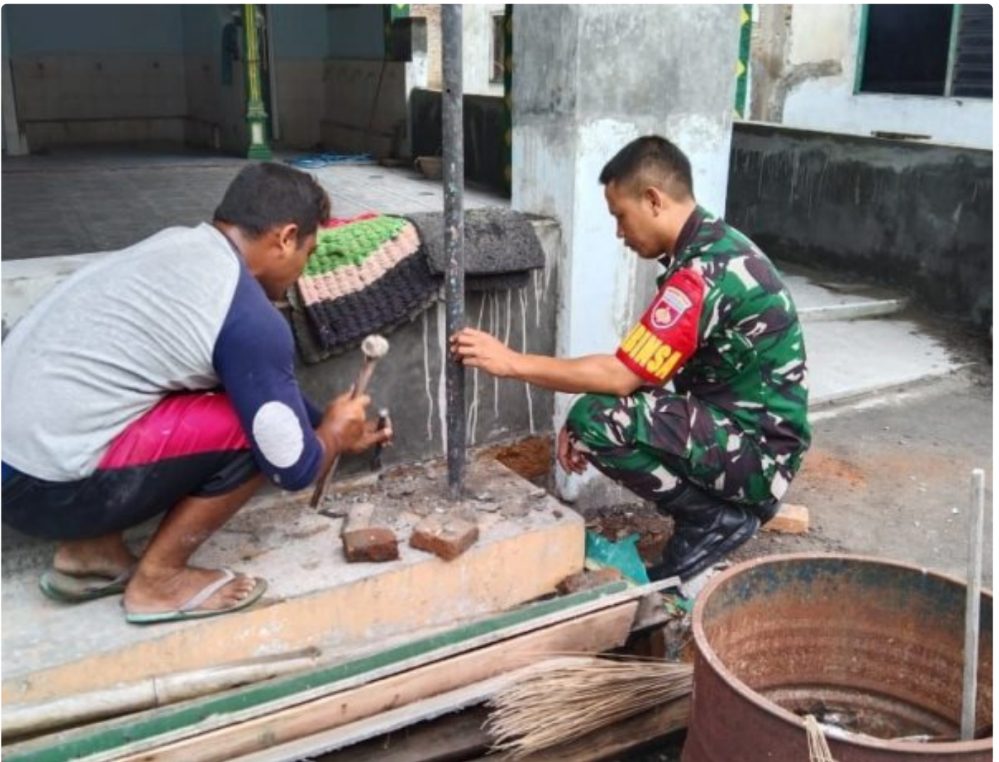
Babinsa Ceper Monitoring Rehab Masjid Di Dukuh Pason
